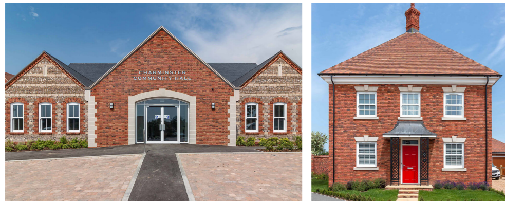
Exemplar homes and facilities delivered by Wyatt Homes.
